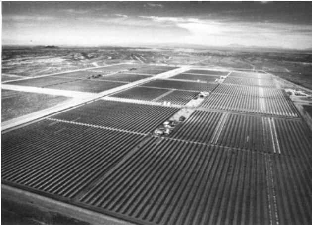
Figure 8.7 The 150 MW solar thermal plant at Kramer Junction, USA. (Source: Solel)
