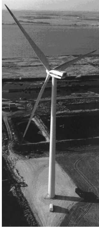
Figure 2.6 The Vestas V90, 3MW wind turbine. (Reproduced with permission of Vestas Wind Systems A/S)
