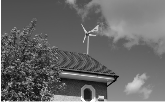
Figure 8.4 Small building integrated wind turbine. (Reproduced with permission of Windsave)
