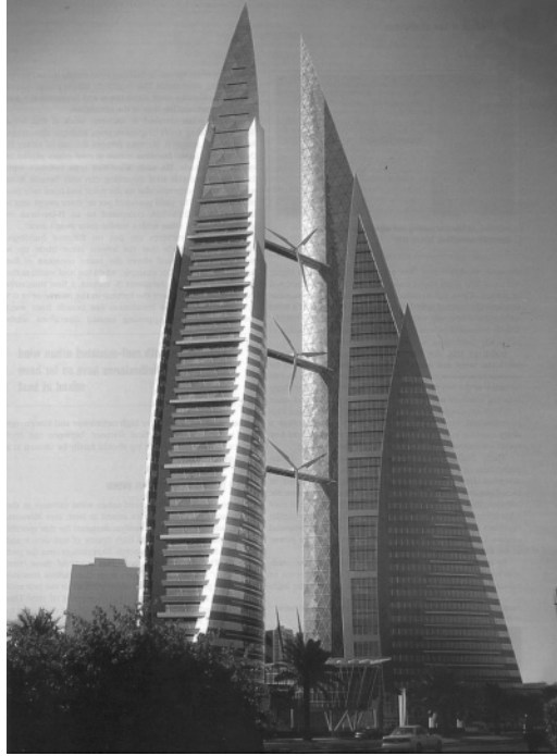
Figure 8.5 The Bahrain World Trade Centre. (Reproduced with permission of the Bahrain World Trade Center image©Khalid Al Muharrqi based on a design by Atkins)
