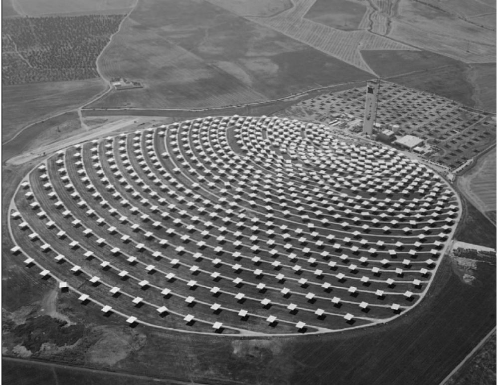
Figure 2.17 Aerial view of 11 MW PS10 solar tower plant at Sanlúcar la Mayor, Spain. (Reproduced from Concentrating Solar Power – from research to implementation. © European Communities, 2007)
